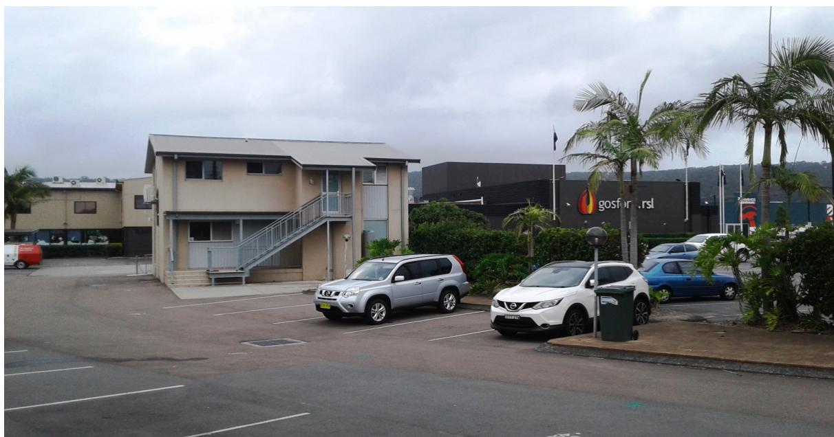
Photo 4 - Hotel Reception Building, looking toward the south-west, 29 Jan 2018.
