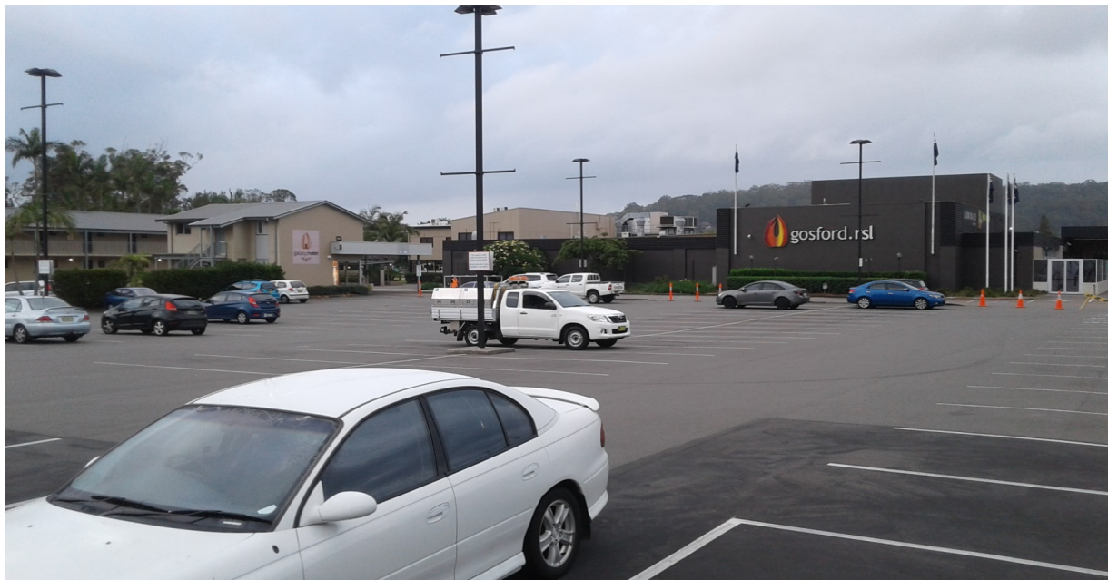
Photo 2 - Site, looking toward the south, existing RSL Club Building at the rear, 29 Jan 2018.
